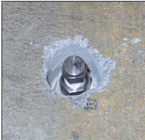
Photograph 4 - Plug and fitting on stainless-steel probe before installation of cement seal
