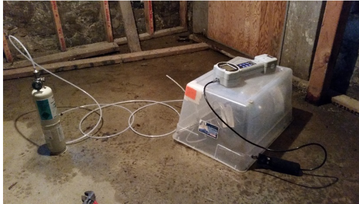
Photograph 23 - Inverted container leak detection method with canister inside of container. Leak detection for vapor point and sample collection apparatus. Helium tank to the left of container.
