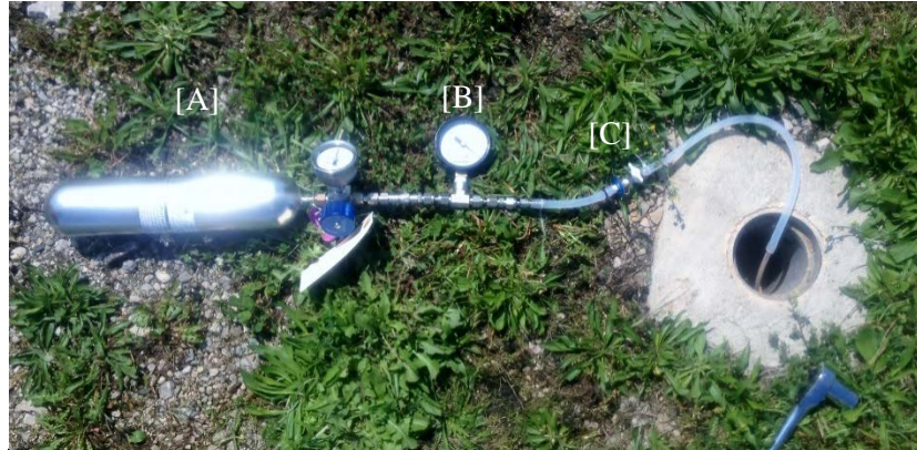
Photograph 13 – Soil gas sample collection set up at deep soil gas vapor point prior to placement of shroud for tracer testing.
