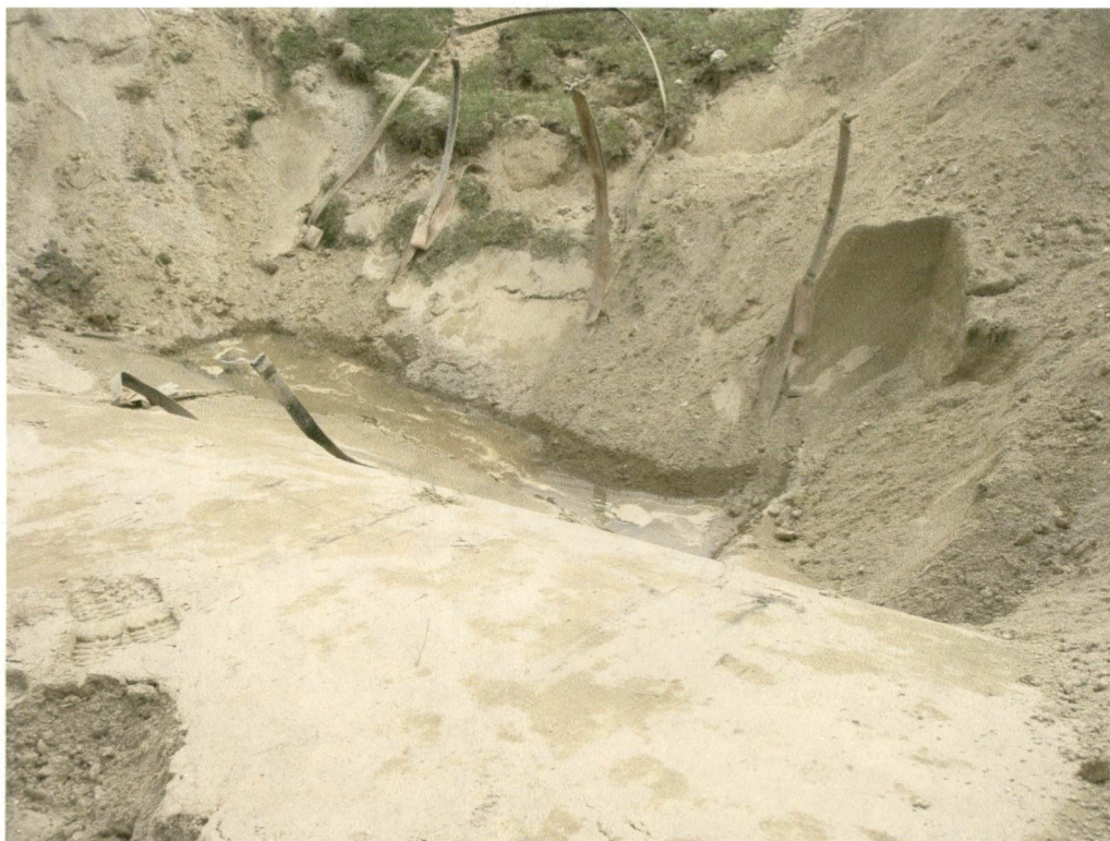
Photograph No. 5 Groundwater in excavation beneath former gasoline UST at CMI Tech Center, Inc. facility (28 July 2008)
